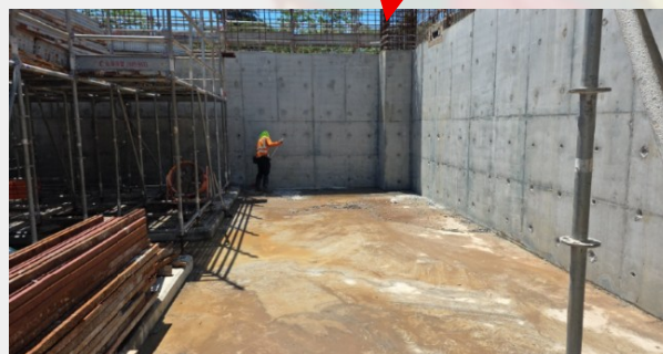
Pumproom and FS Pumproom Superstructure Construction in Progress 泵房及消防泵房大樓結構工程進行中
