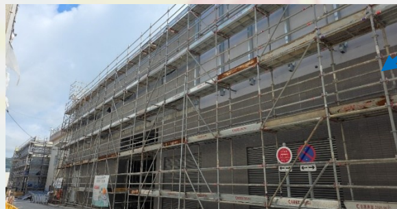
Tiling works for external wall of MBR Treatment Facilities in Progress 薄膜生物反應處理大樓的外牆磁磚鋪設 工程進行中
