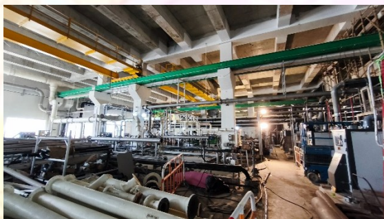
Process Equipment Installation at Membrane Bio-reactor Treatment Facilities in Progress
