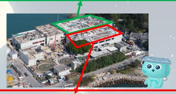
Superstructure Construction at Preliminary Treatment Facilities Completed and E&M Installation In Progress
