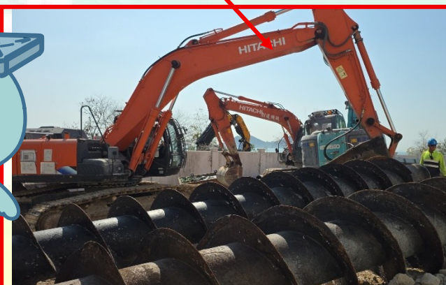
Demolition of the existing Screw Pump House in progress 拆除現有螺桿泵房進行中
