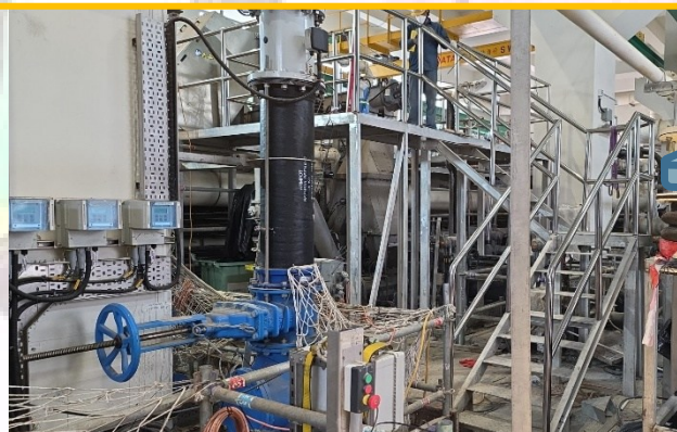
Installation of steel platforms at Preliminary Treatment Facilities in progress 基本污水處理大樓工作平台安裝工程進行中
