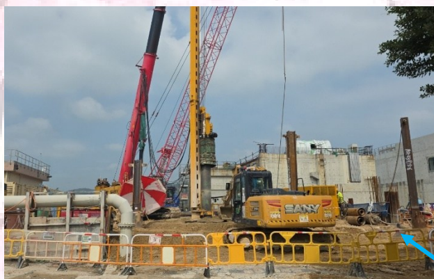
Piling works for Sludge Centrifuge House in progress 污泥離心機大樓的樁基工程進行中
